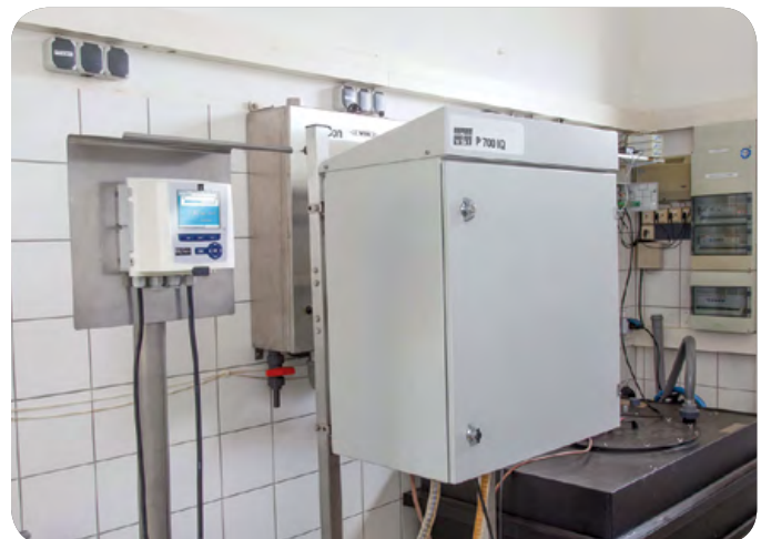
System 282/284 with Orthophosphate analyzer P700 IQ
